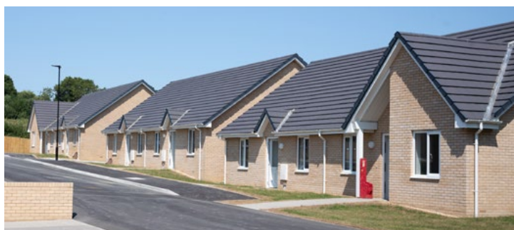
Ryde, Isle of Wight – under construction
